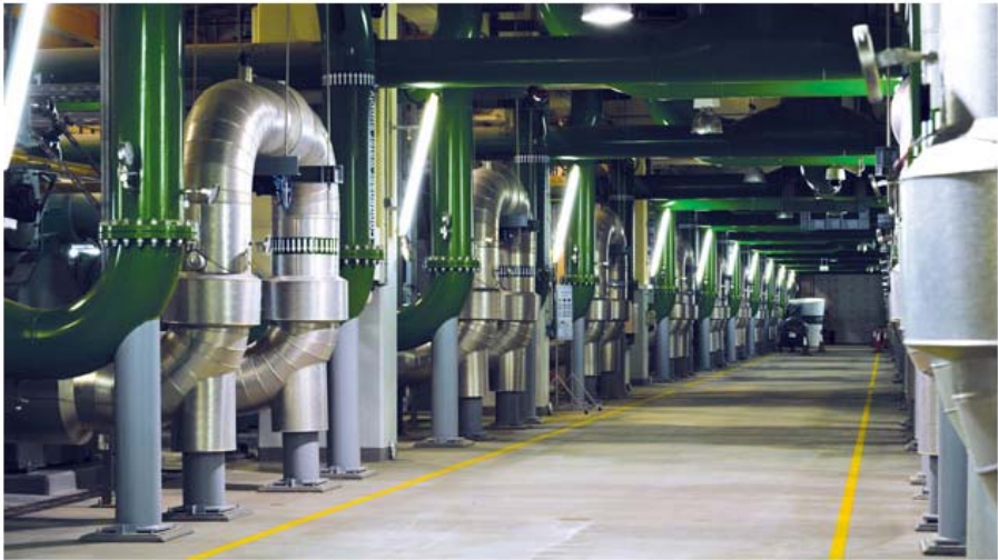
Chiller room inside the largest district cooling plan in the world, at The Pearl-Qatar. (Image courtesy Qatar Cool)
