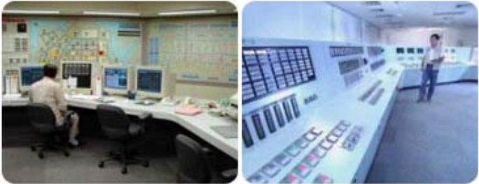
(DCS central chiller plant control room)
